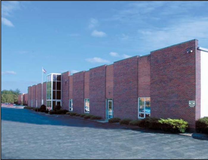
Kirkwood, Missouri USA Manufacturing Plant
